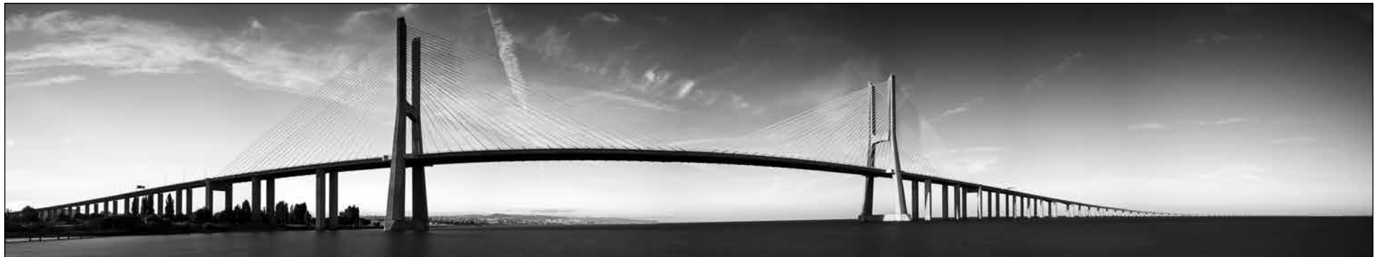
E-vasco de gama bridge
